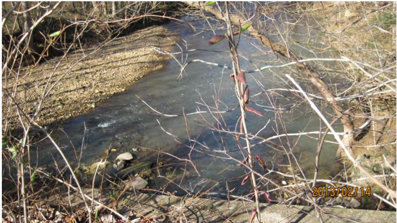
Photo 1. Downstream view of STR-1 (Summers Branch) taken from existing I-65 box culvert.
