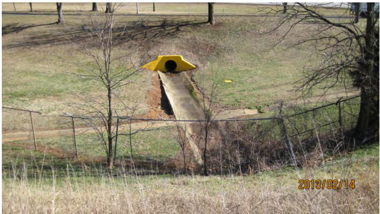
Photo 4. Up gradient view of WWC-1 taken North of Lake Springs Road.
